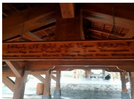
Figure 7. The Second Stairway
