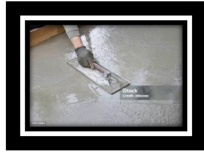
Gambar 4. Concrete Screed Sumber: Goggle
